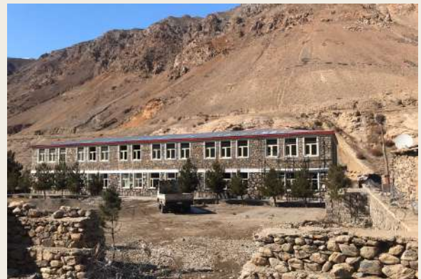
2019 / 2020 Mixed secondary school in Dahan e Rewat
